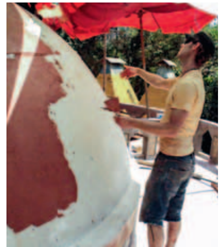
Clockwise from above left: Detail of the tadelakt surface at the top of the dome; the final colourful and glossy result is much admired; the area was wet down and shaded to aid slow curing; applying the tadelakt coating required some agility.
