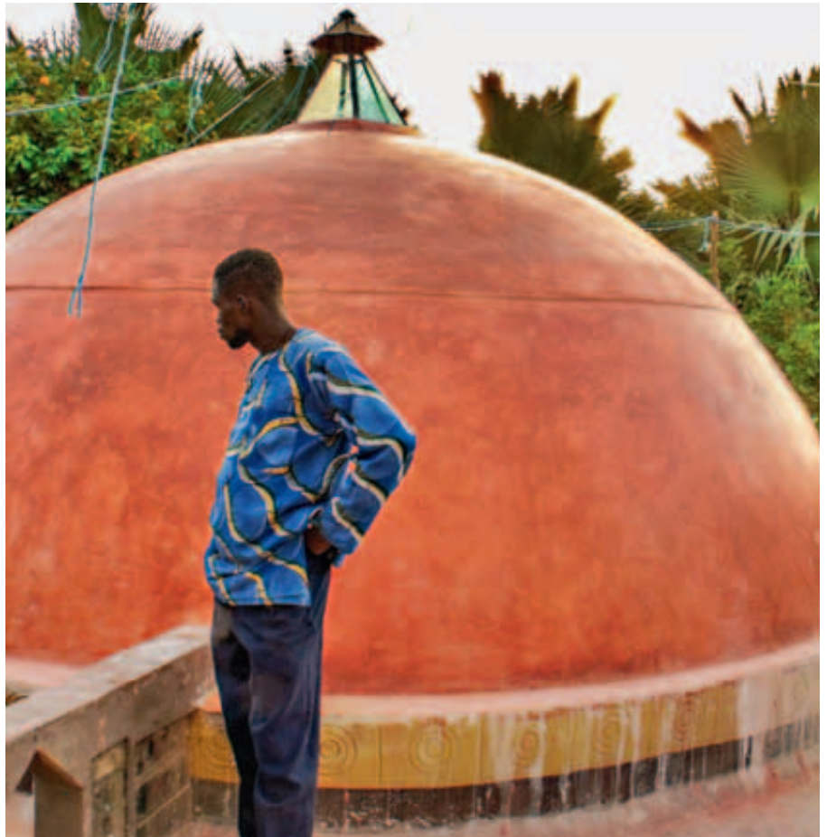
Clockwise from above left: Detail of the tadelakt surface at the top of the dome; the final colourful and glossy result is much admired; the area was wet down and shaded to aid slow curing; applying the tadelakt coating required some agility.
